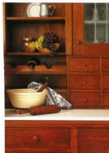
▲ THIS COLONIAL-STYLE HUTCH IS BUILT FROM HAND-PLANED PINE THAT'S STAINED A WALNUT COLOR. THE CABINET CASE IS FACE-FRAME, AND EACH DRAWER IS INSET INTO THE FACE FRAME. THE OUTSIDE EDGE OF THE CABINET IS BEADED, AND SHELVES HAVE MULTIPLE BEADS FOR A SUBTLE CONTRAST.
