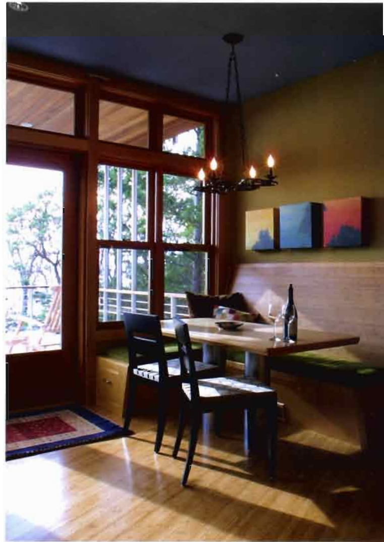
THIS ONE-SIDED BANQUETTE WITH MOVEABLE SEATING provides dining space in a small getaway house. The tabletop—supported by two pedestals and a plate of sheet steel—is rigged to slide away from the banquette to make it easy for anyone to get in and out. The bench provides a storage drawer on one end.
