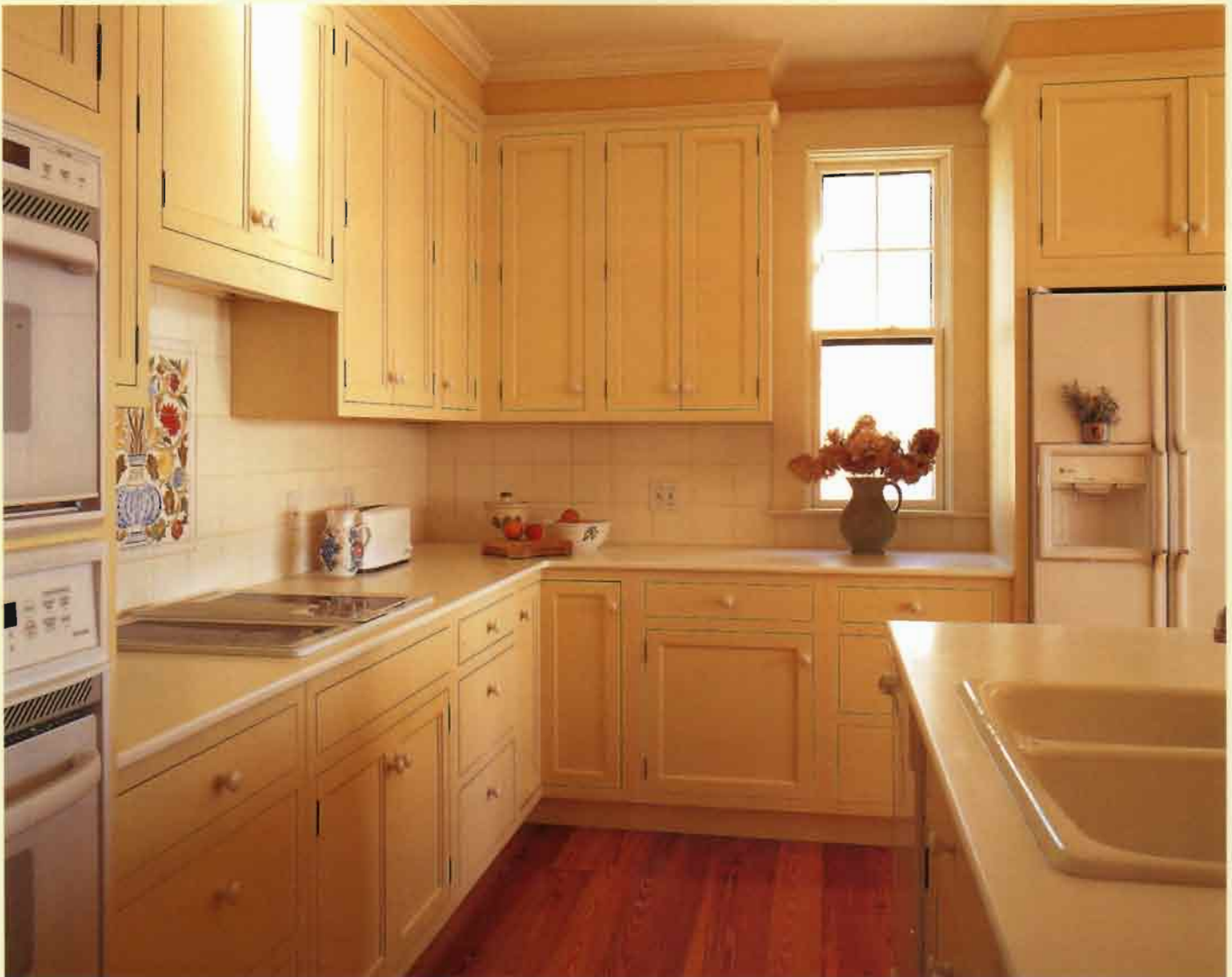
▲ A WHITE SOLID-SURFACE COUNTERTOP WITH EASED EDGES brightens an urban kitchen that has only one window. Flat white 4-in.-square tile makes a water- and heatproof backsplash. The space between the cabinets is filled with flat trim topped with crown molding and painted a darker gold to match the softwood floor.
