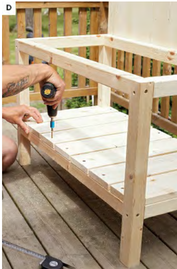
D. Screw on the planks for the bottom shelf.
