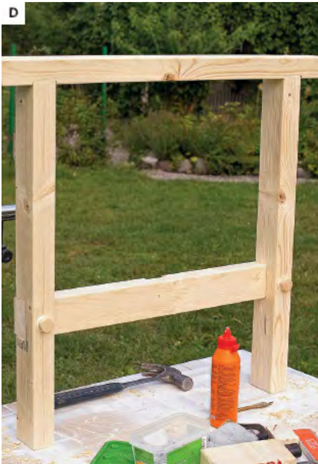
A–D. Start by building the legs, which consist of two lumber upright posts with an inserted crosspiece. Mark the area where the crosspiece is to go onto the legs. With a
