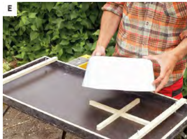
E. Now it's time to make the mold for casting the concrete work surface. I like to use shuttering plywood for my mold. Saw pieces to make a small, shallow box. I used the same kind of tub that will be used later to make the tub hole in the concrete, and cut off its upper rim. The tub is secured by weighing it down with a few stones and a simple cross inside the mold—the tub must not move when the concrete is poured into the mold.
