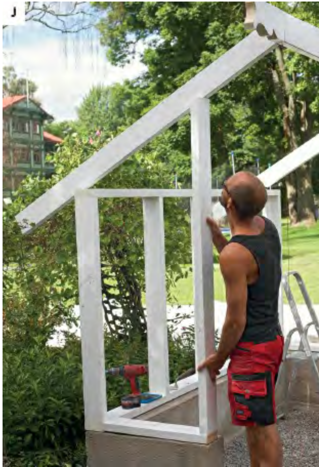
J. The short side frame is built in place.
