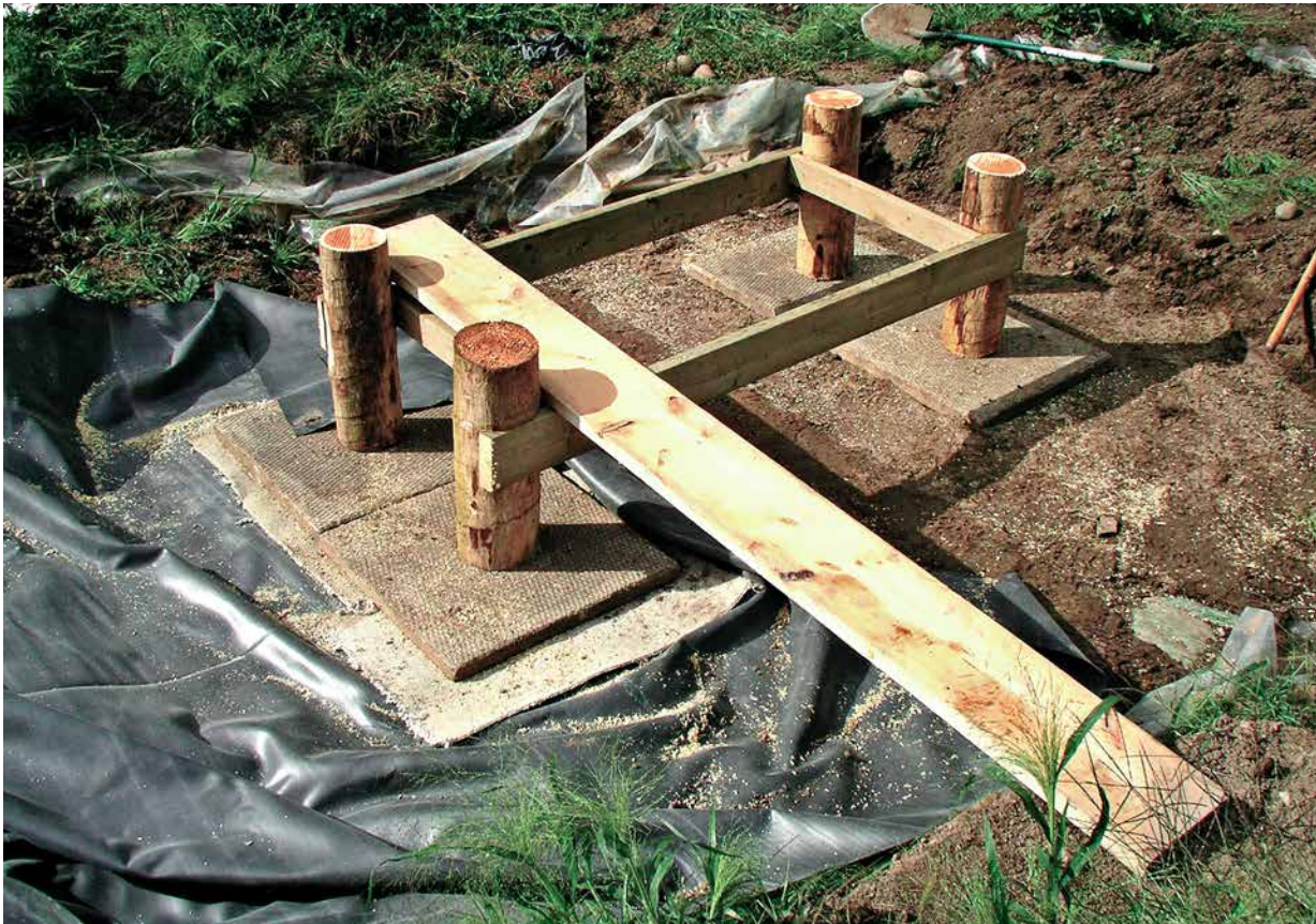
FIGURE 22 Footings for the bridge shown in figure 13.
