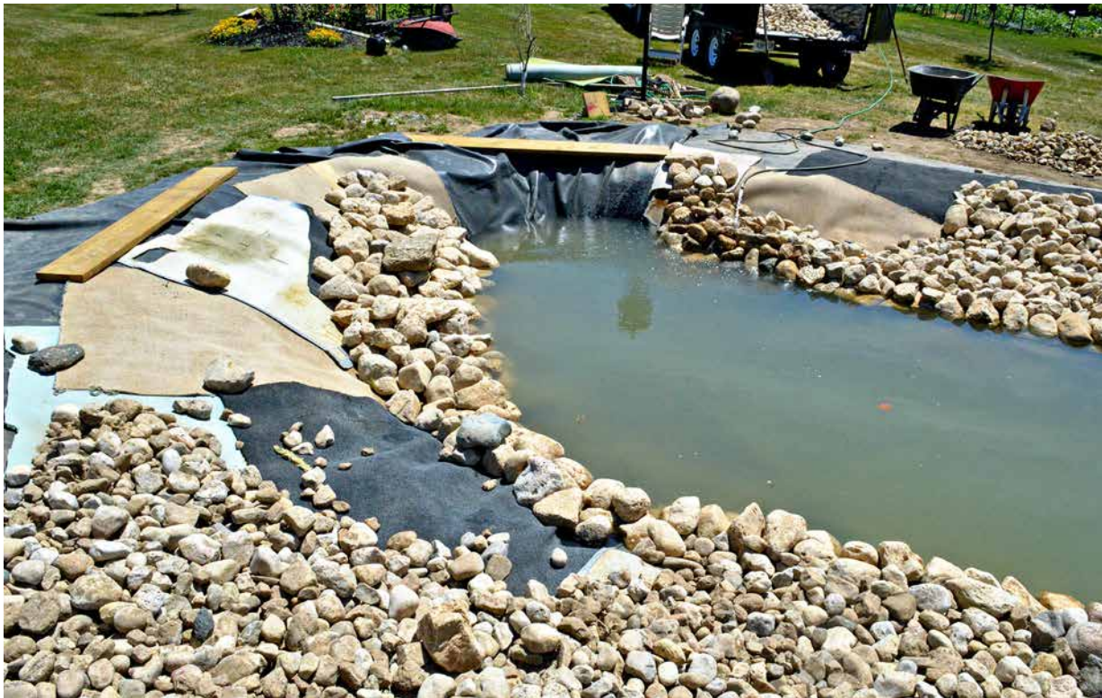
FIGURE 23 Carpet has been used as the overlayment to prevent punctures from above the liner.
