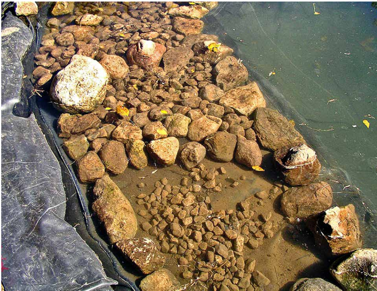
FIGURE 25 Partially completed planting shelves.
